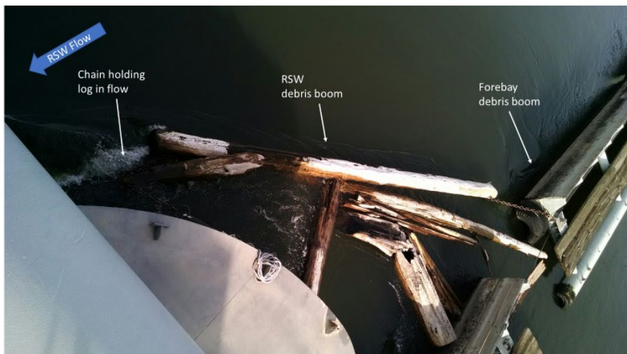
Photo 1. Forebay south side of RSW.
